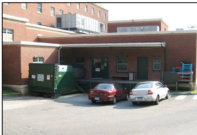
McConaughy Hall Service Area and Loading Dock
