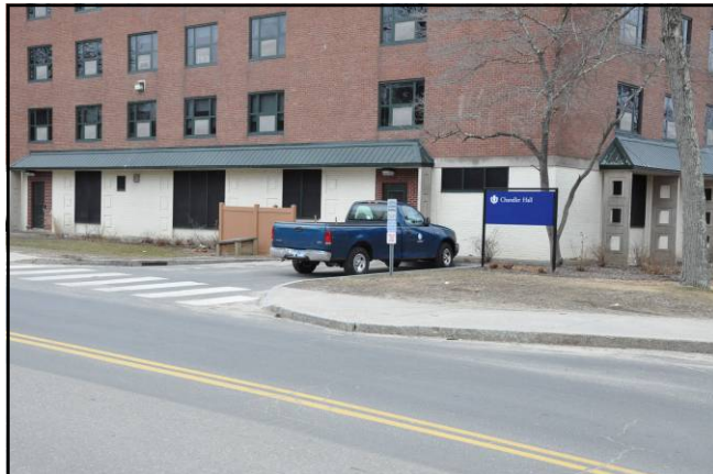
Access to Chandler Hall Service Area from Gilbert Road.
