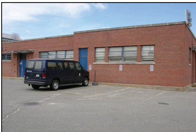
Service parking and Service Area at Athletic Facilities Building.
