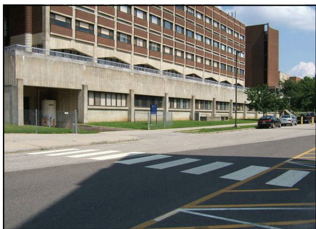
Physics Building on Auditorium Road.
