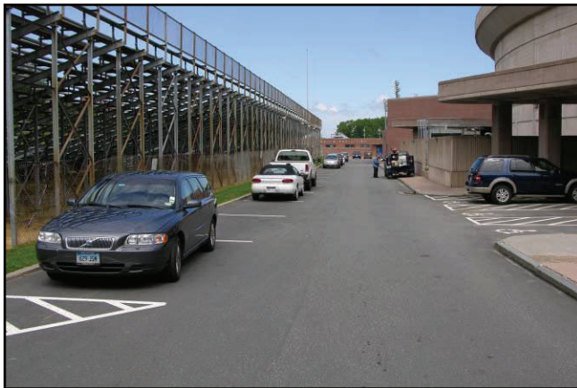
Access Road from Stadium Road to Athletic Facilities Bldg.
