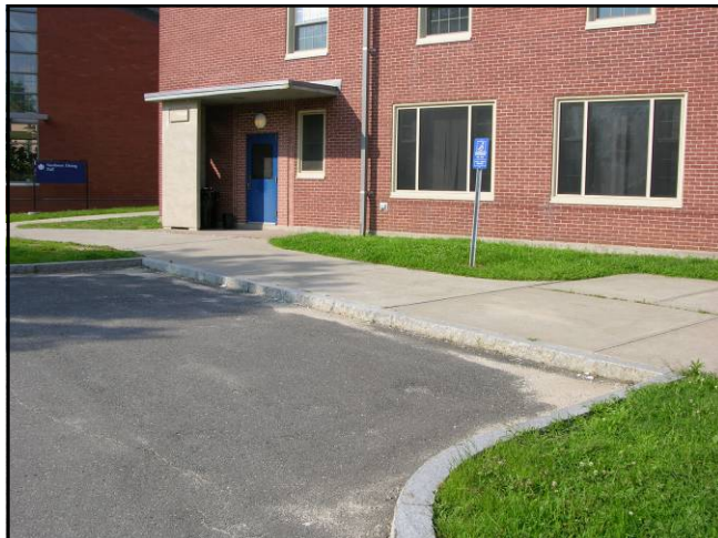
Terry Hall Service Area.
