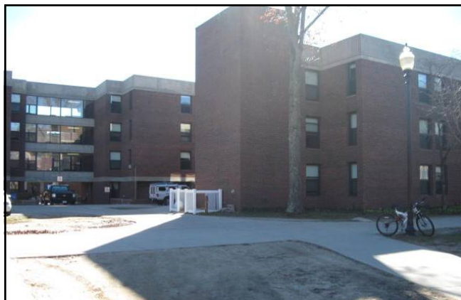
Sidewalk leading from School of Business Service Area to Graduate Residences A-B Service Entrance.
