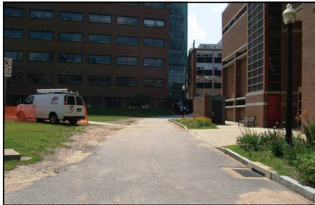
Access Road to Pharmacy/Biology Service Area.
