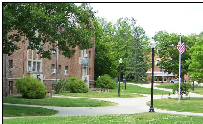
Sidewalk from CUE Service Area to Koons Hall, past the Hall Building on left and beyond the flag pole.
