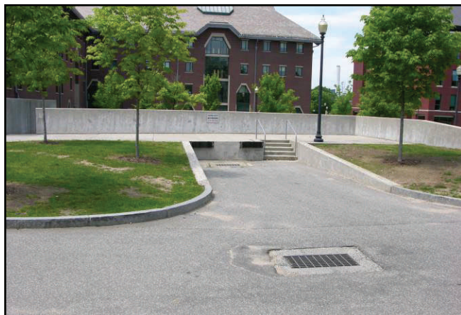
Loading Dock at the School of Business.
