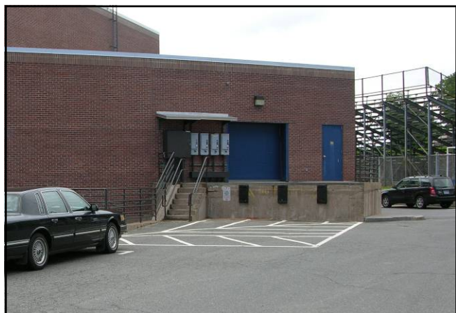
Loading Dock at back of Gampel Pavilion.
