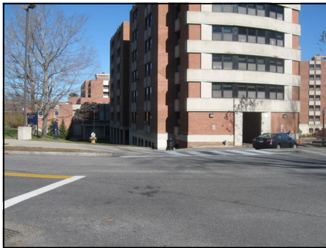
Entrance to Brock Hall service area.
