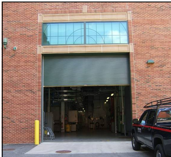
Overhead door on the east side of the Chiller facility.
