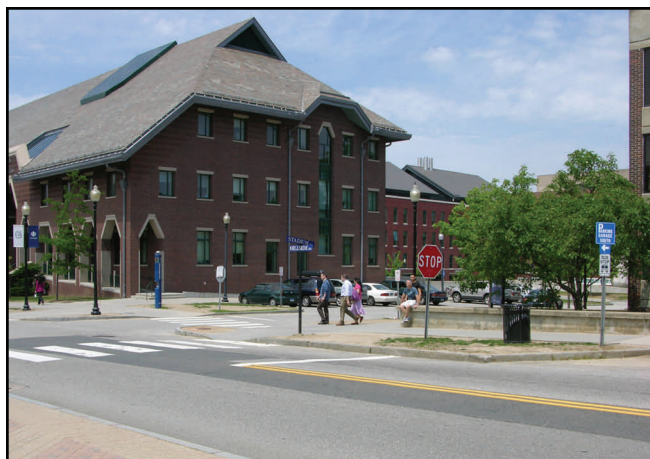
Intersection of Hillside Road and Stadium Road to the School of Business Loading Dock.
