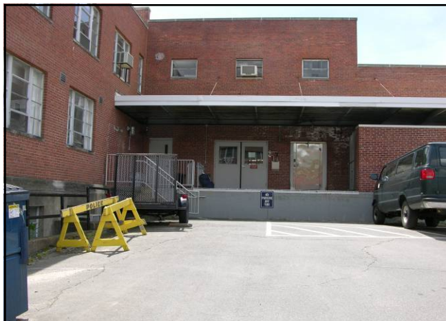
Service Area and Loading Dock of White Building and Dairy Bar.
