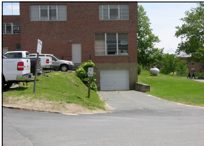
Service Area of Jones Building
