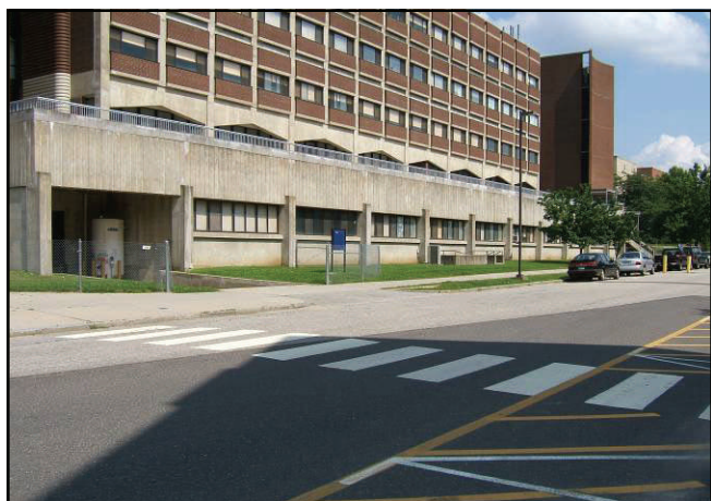
Physics Building on Auditorium Road.
