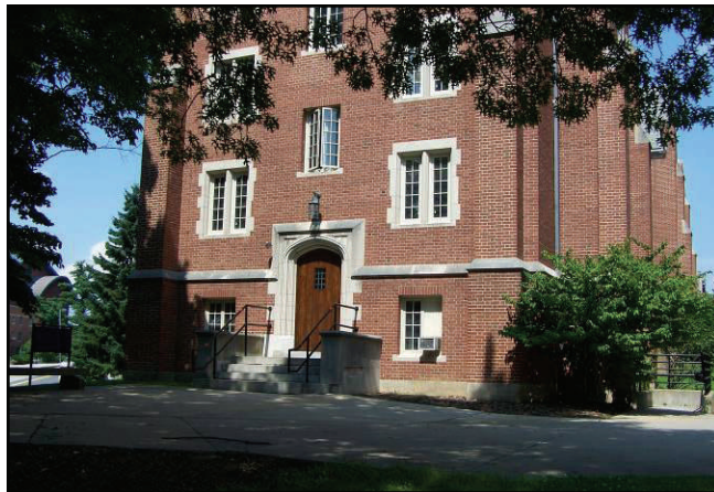
West entrance to Wood Building.
