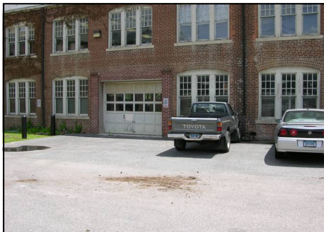
Service Area for Klinck Building
