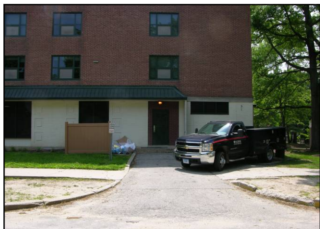
Service Area at Alsop Hall
