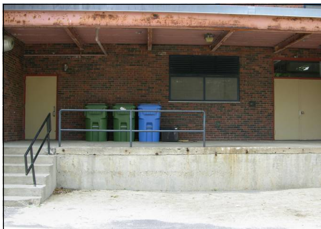
Buckley Loading Dock
