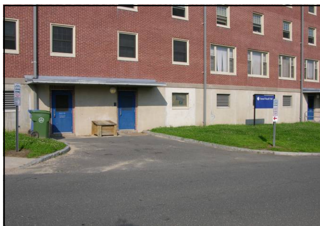
Russell Hall Service Area.
