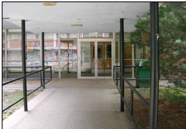
Service route to the entry door at Schenker Hall.
