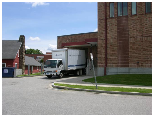
East loading dock at the Ag-Bio building.
