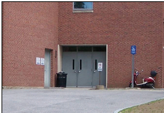
Service Area and building service entrance.
