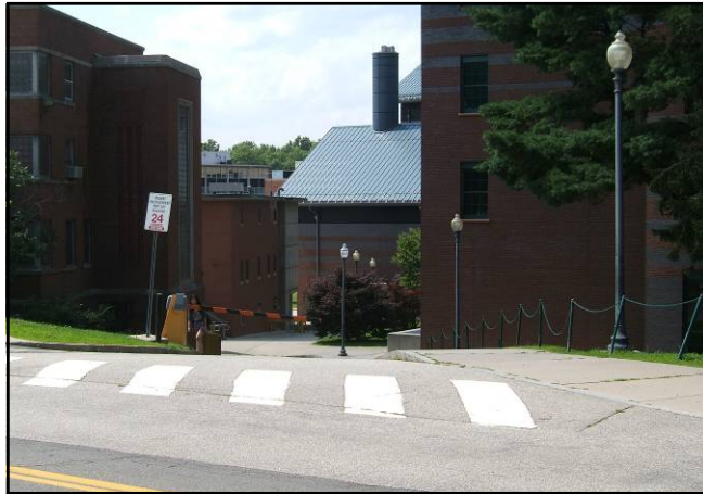
Access Road from behind Chemistry.
