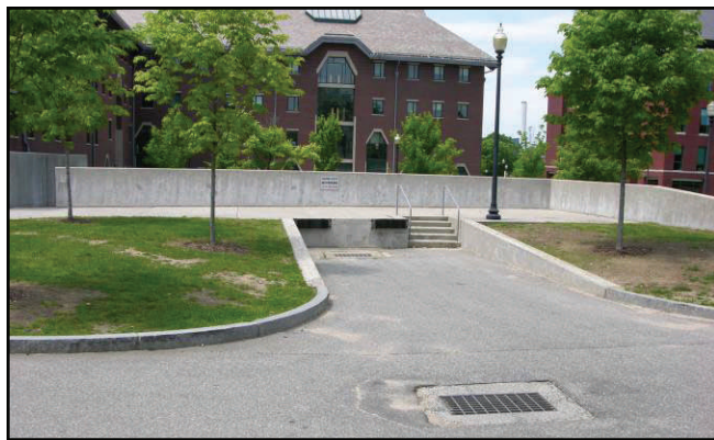
Loading Dock at the School of Business .
