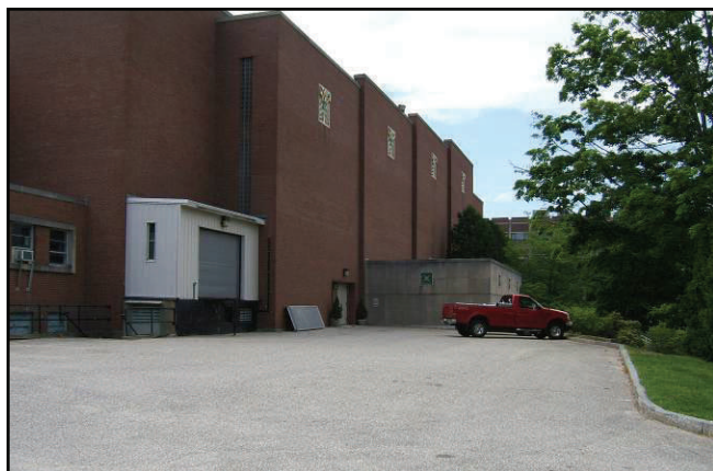
Jorgensen Center Service Area and Loading Dock.
