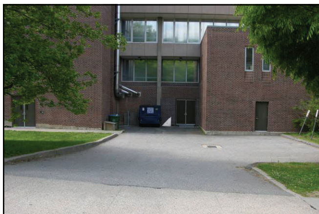
Bousfield Loading Dock and Service parking spaces.
