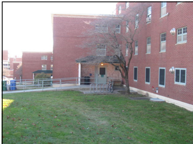
The Litchfield Service Entrance.
