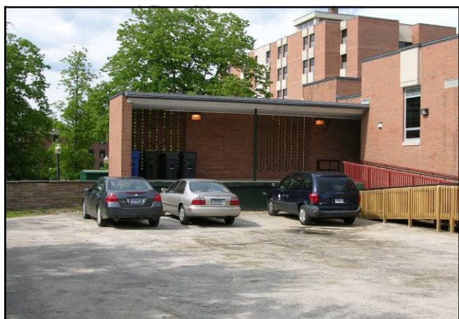
The Service Area and Loading Dock at Ryan Refectory.
