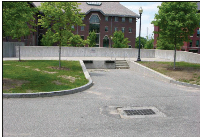
Loading Dock at the School of Business.
