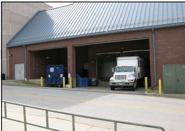
UConn Co-op Loading Dock
