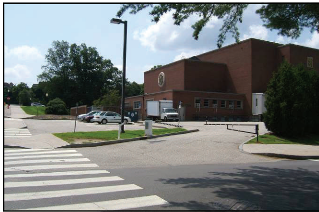
Entrance to Service Area at corner of Glenbrook and Jorgensen Roads.
