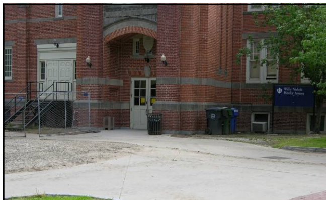
Service Doors at Hawley Armory.
