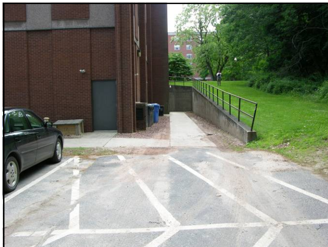
Path to loading doors at Bishop Center
