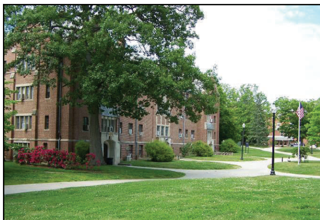
Sidewalk access from the Service Area at the CUE to the front doors of the Hall Building.
