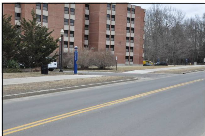
Entrance to Ryan Refectory Service Area from Hillside Road.
