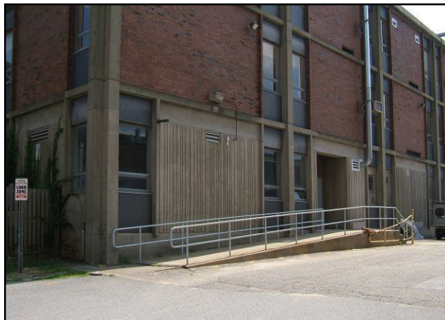
Ramp to Service Doors of Bronwell.
