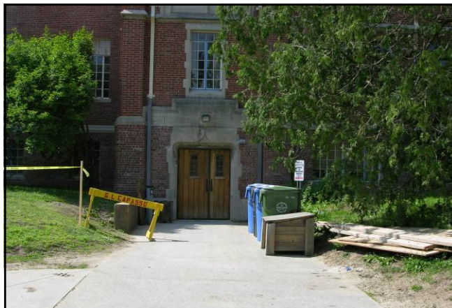
Loading Doors of Family Studies Building.
