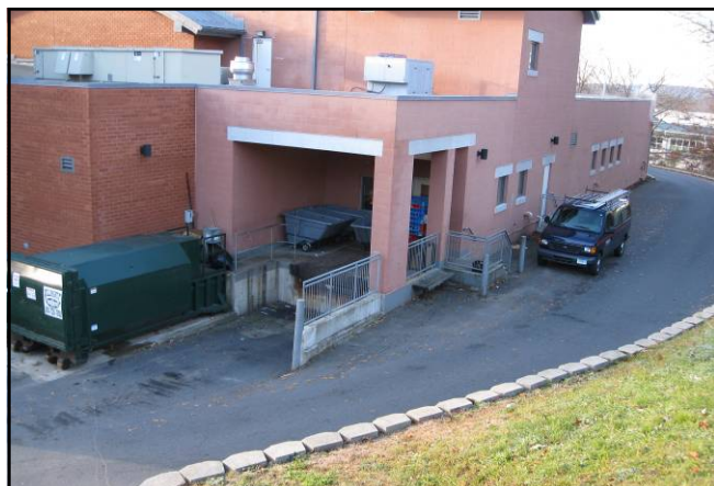
Loading Dock at Northwest Dining Hall.
