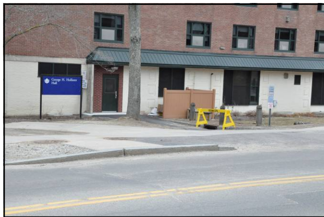
Hollister Hall Service Area from Hillside Road.
