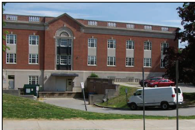
Wilbur Cross Building Loading Dock.
