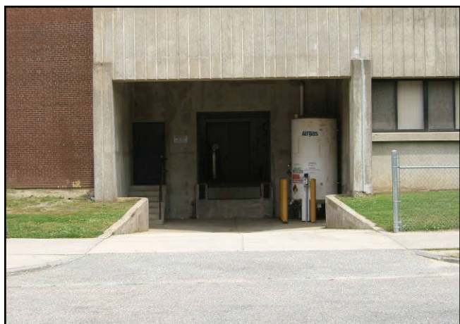
Loading Dock at Physics Building.
