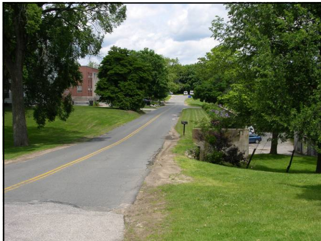
Access Road to Jones Building
