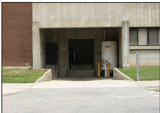
Loading Dock at Physics Building.
