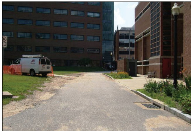
Access road to Torrey Service Area.
