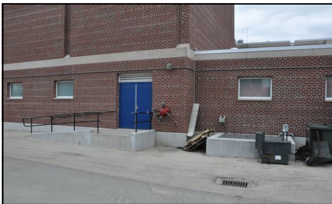
Physical Education building service entrance.
