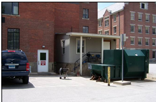
Service door located on northwest corner of Whitney Hall.
