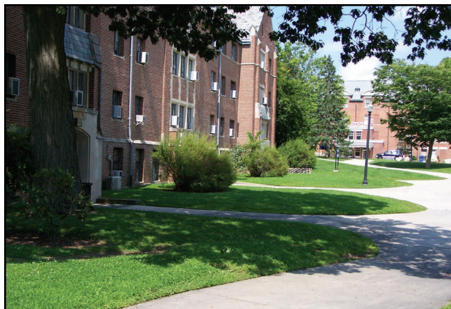
Front doors to Hall Building.
