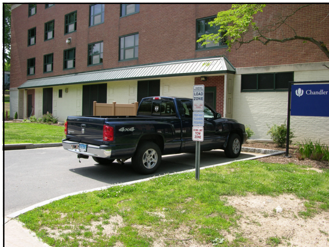
Loading zone for Lancaster Hall.
