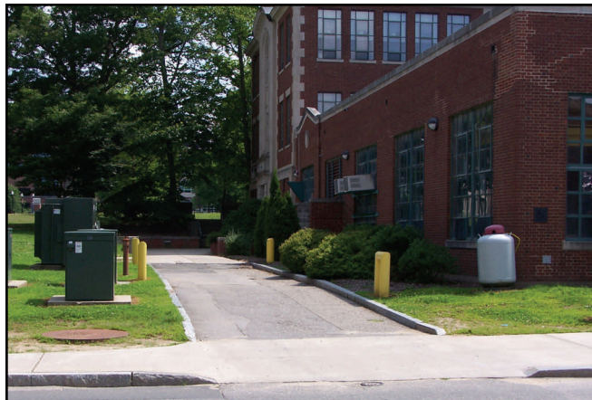
Service Area on east side of Castleman off Glenbrook Road
