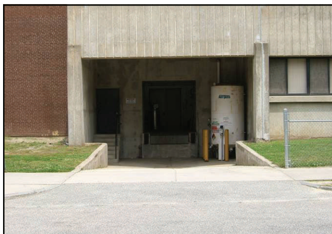
Loading Dock at Physics Building.
