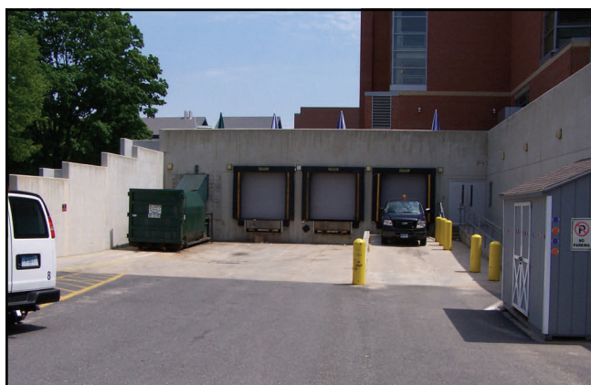
Student Union Loading Dock with internal service corridor.
