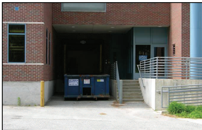
Loading Dock of Dodd Research Center
