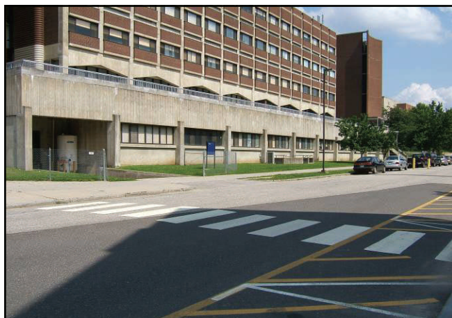
Physics Building on Auditorium Road.
