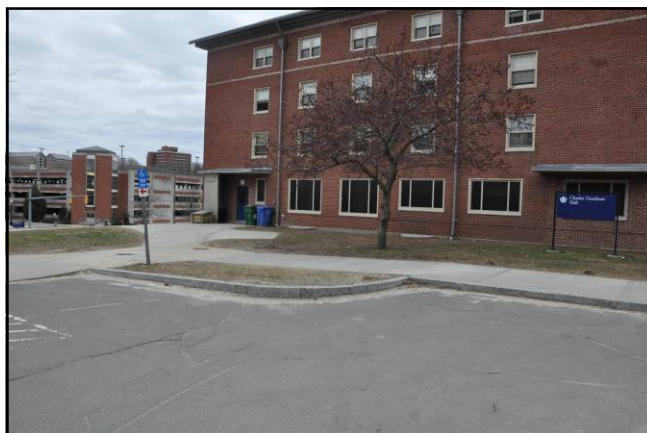
Goodyear Hall Service Area and entrance.
