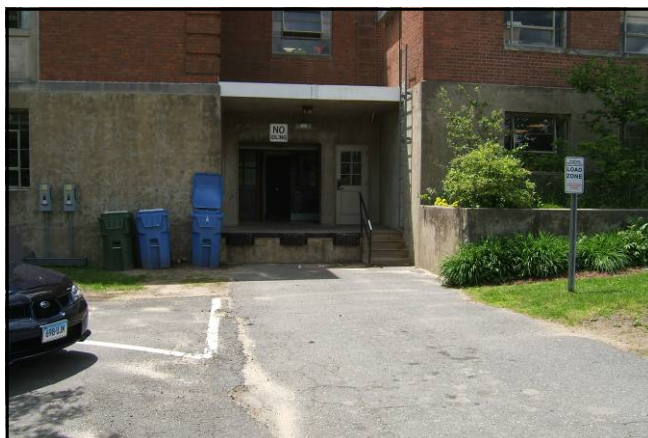
Loading Dock of Young Building
