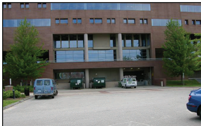
Babbidge Library and Loading Dock.
