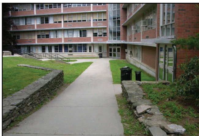
Sidewalk from Whitney Road to Monteith door.
