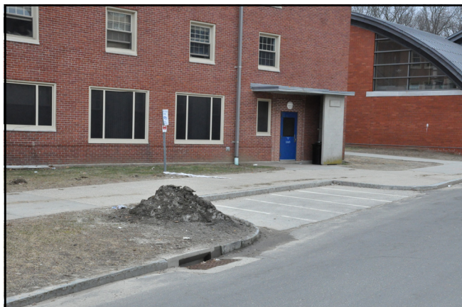
Rogers Hall Service Area and entrance.
