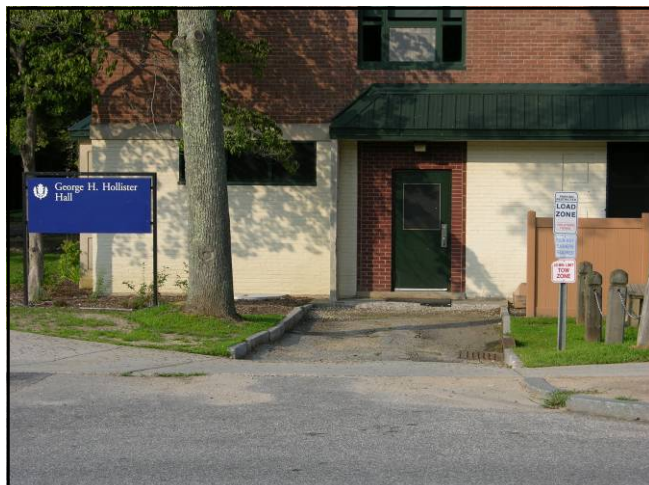
Hollister Hall Service Area.
