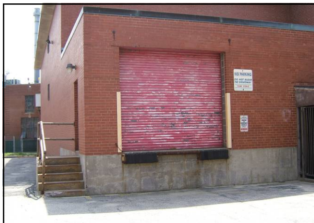
Loading Dock at Central Recycling & Storage building.
