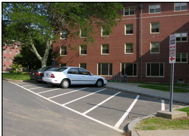
Batterson Hall Service Area.
